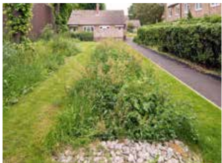
A swale at Queen Caroline Estate in West London, part of Groundwork's LIFE+ climate-proofing project
